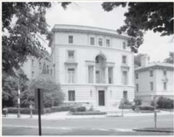
Joseph Beale House, 2201 Massachusetts Avenue, N.W., Washington, DC, 1907-1908. Glenn Brown, Architect. (J. Alexander, Photographer, 1971, HABS)
