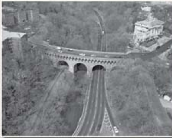
Dumbarton Bridge (Buffalo Bridge), 1913. Glenn and Bedford Brown, Architects. (Jack Roscher, photographer, IABR 1993) Brown designed the Dumbarton Bridge, known colloquially as the Buffalo Bridge, with his son and partner Bedford Brown, IV. This masonry bridge displays the heavy stone and semicircular arches ingrained while working on A.L.I. Richardson's project many years ago. The bridge is unusual in that it carries an accommodated Q Street, NW over Rock Creek Park between 18th century Georgetown and the rigid geometry of the Washington street grid. Above the five arches are 56 carved Indian heads and the entrances are flanked by stylized trees.
