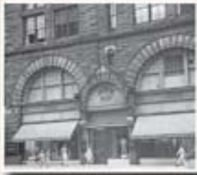
Cheney Building, Hartford Connecticut. Henry Hobson Richardson, Architect, 1875. (Photo: Constance Layton, Connecticut Historical Commission, July 1970) This building is a powerful composition of granite and ironstone, with semi-circular arches and roughly cut stone emphasizing the building's mass. Brown became Clerk of the Works for the construction of the Cheney Building and worked on it for two years until it was completed. By the time he left Hartford, Brown was extremely familiar with the design and construction of Richardsonian Romanesque style buildings. Not surprisingly, much of Brown's early work in Alexandria, both residential and commercial, shows the unmistakable influence of his training while working on this building.
