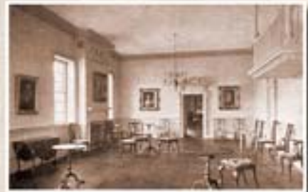
Gaddy's Tavern Ballroom (Alexandria Special Collections) Nearly two decades after his initial recording of the building's woodwork, Glenn Brown remained intensely interested in the fate of Alexandria's colonial architecture. By 1897, the venerable Gaddy's Tavern, the setting of balls for George and Martha Washington, Thomas Jefferson's first inaugural party, and many other significant events, had fallen into a deplorable condition. Brown learned that the Metropolitan Museum of Art was buying examples of American architecture for its forthcoming American Wing, and mounted an effort to save the ballroom woodwork by having the museum acquire it. In the 1890s, renowned restoration architect Thomas Eliason Waterhouse traveled to New York to take measurements of the original woodwork in order to create the replica ballroom which visitors to Gaddy's Tavern see today.
