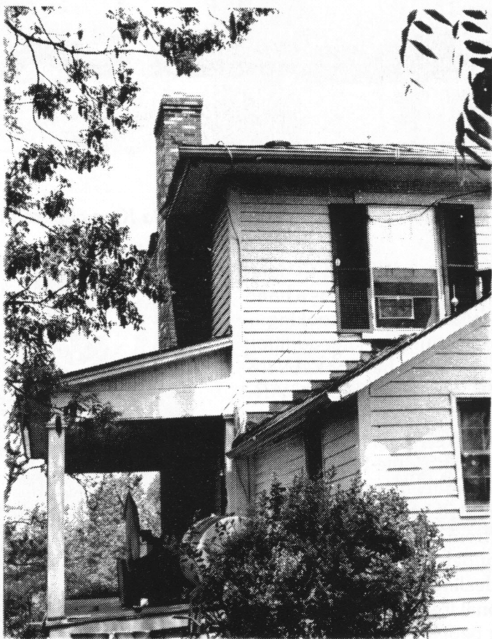
Older section of "Cap" King's house, with added kitchen, foreground
