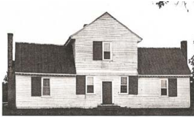
Fig. 17. Azariah Graves House. Handsome three-part Georgian-style house built by one of Yanceyville's patriarchs.
